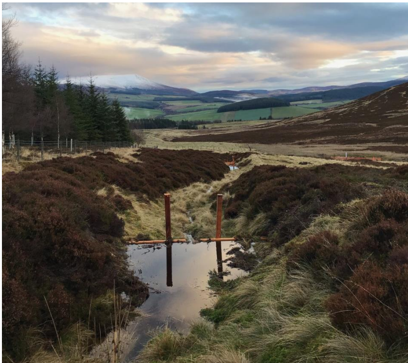
Figure 1: An example of Nature Based Solutions at Glenlivet, NE Scotland. Timber dams designed to slow the flow, store runoff and replenish groundwater storage.
